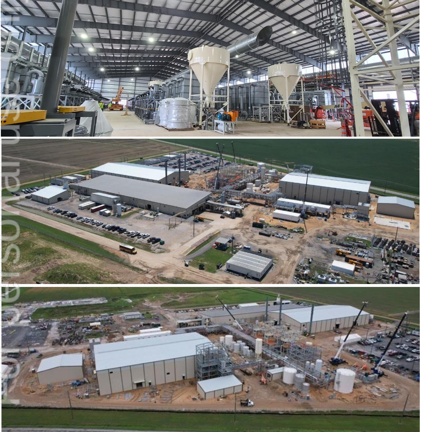
Figure 2: Construction of 11.25ktpa AAM Vidalia facility.
