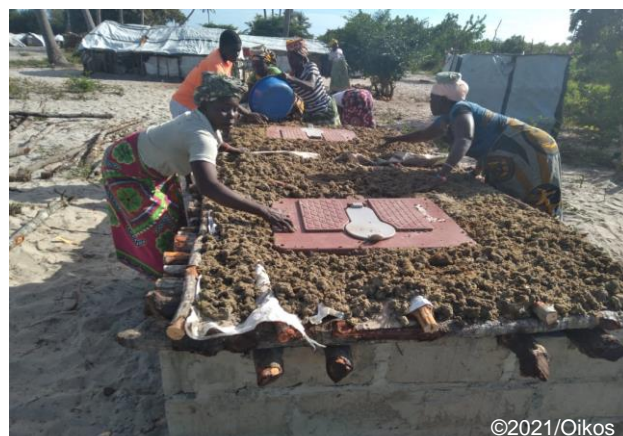
Building elevated emergency latrines on Ibo Island due to sandy soil
