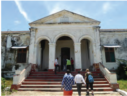
178_Buffer zone_Primary school.JPG
