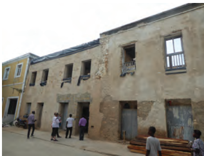
022_Stone and lime town_Building under intervention.JPG
