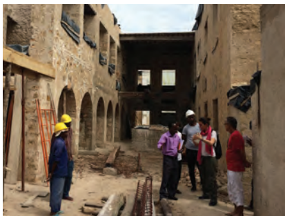
025_Stone and lime town_Building under intervention.JPG
