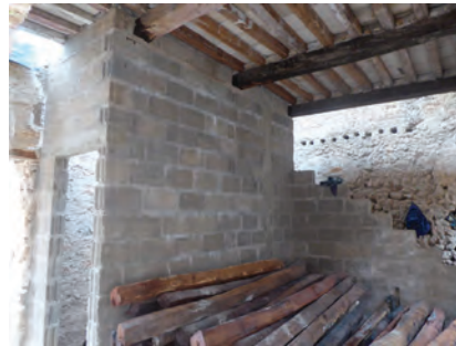
026_Stone and lime town_Building under intervention.JPG
