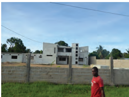
186_Buffer zone_Moz.Island continent_new house.JPG
