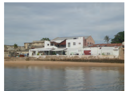
199_Island seafront_Change of the seafront façades.JPG
