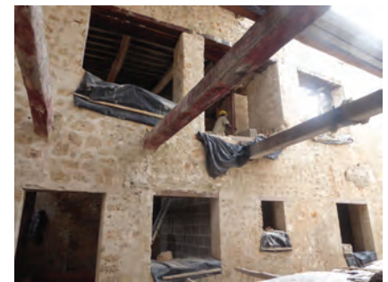
024_Stone and lime town_Building under intervention.JPG
