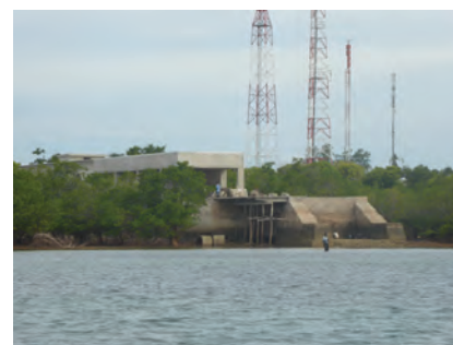
158_Unpermitted construction_site A.JPG
