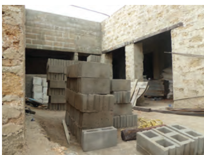
028_Stone and lime town_Building under intervention.JPG
