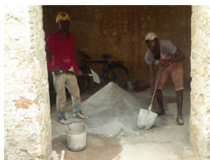
029_Stone and lime town_Building under intervention.JPG
