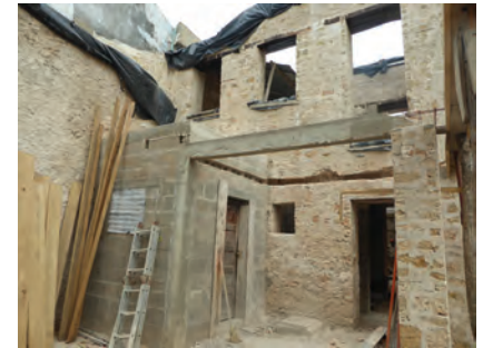
027_Stone and lime town_Building under intervention.JPG
