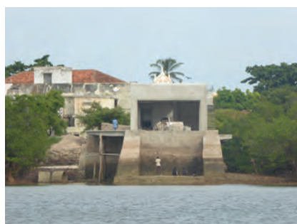
159_Unpermitted construction_site A.JPG
