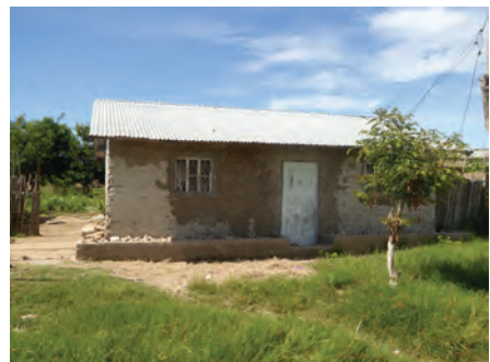
185_Buffer zone_Moz.Island continent_state house to remove people from island.JPG
