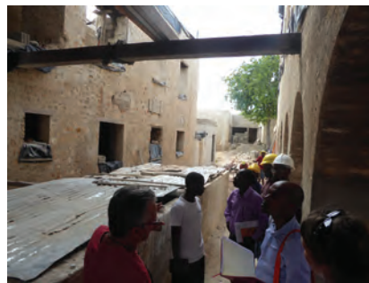
023_Stone and lime town_Building under intervention.JPG
