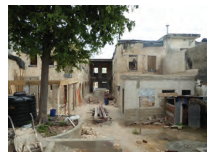
030_Stone and lime town_Building under intervention.JPG
