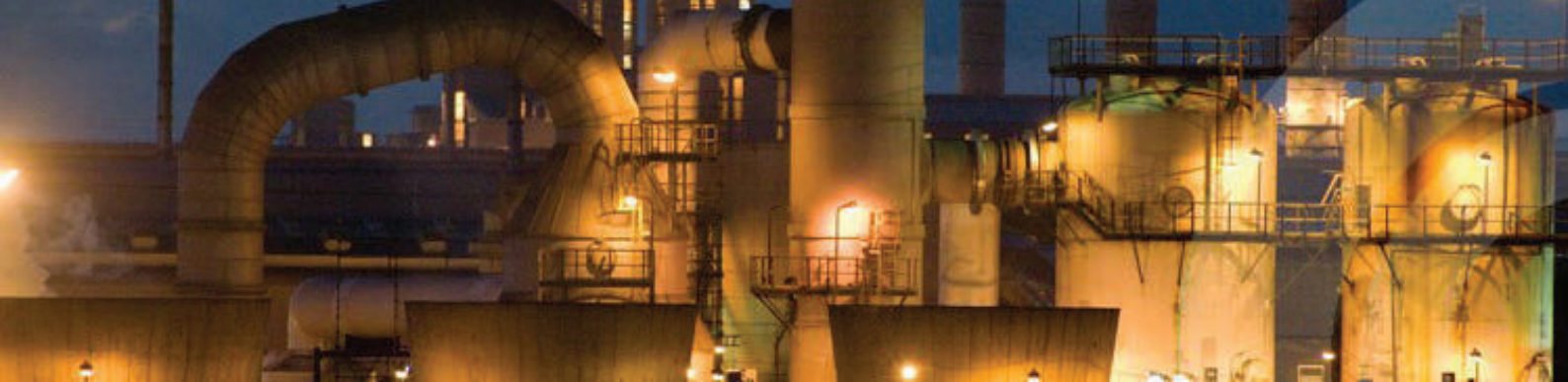
The Foskor terminal at the Richards Bay port in South Africa (source: Foskor)
